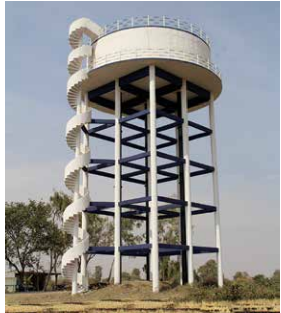
360 KL Capacity Break Pressure Tank for Buldhana Water Supply Scheme, in Maharashtra
