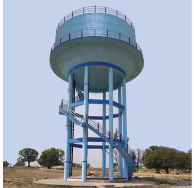
400 KL Overhead tank for Kandaila Multi village Rural Water Supply Scheme in Rewa district, in Madhya Pradesh.
