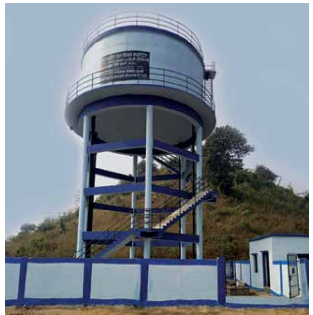
240 KL Overhead Tank staging 12 mtr at Village-Jajagarh, for Indwar-I Multivillage Rural Water Supply Scheme in Umariya and Katni District, in Madhya Pradesh.
