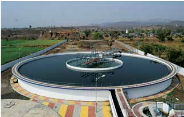
31 MLD Water Treatment Plant at Jalgaon Jamod for Maharashtra Jeevan Pradhikaran, in Maharashtra.
