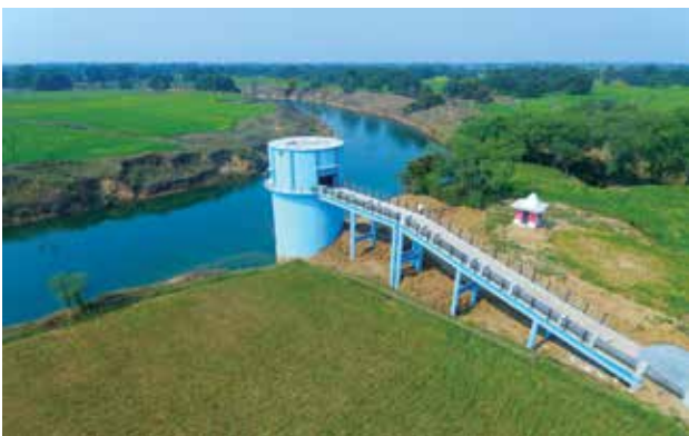
Intake well cum pump house for Kandaila Multi village Rural Water Supply Scheme in Rewa district, in Madhya Pradesh.
