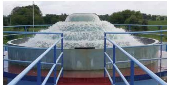
Cascade Aerator of Bankpura WTP of capacity 14.75 MLD at Kandiyakhedi, Block Bairaora, Dist Rajgarh. In Madhya Pradesh.
