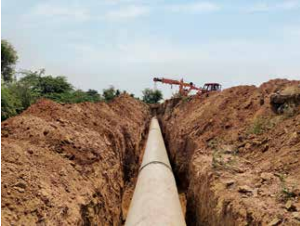
1067 mm dia MS pipeline laying for Madurai package-1, in Tamil Nadu.
