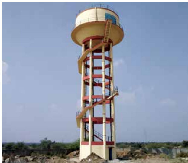
300 KL 20 mtr. Staging OHSR at Ganderi under Kishangarh Cluster of Jahazpur Project, in Rajasthan.
