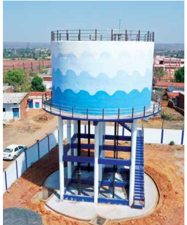
300 KL Overhead Tank staging 9 mtr at Tendukheda Town, for Bhedaghat Water Supply Scheme, in Madhya Pradesh.
