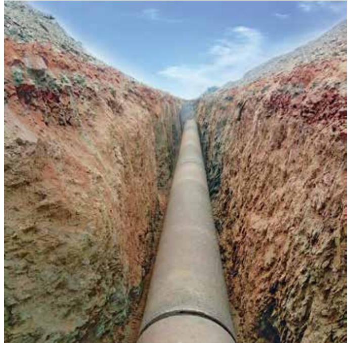
800 mm dia MS pipeline laying at Jahazpur Project, in Rajasthan.
