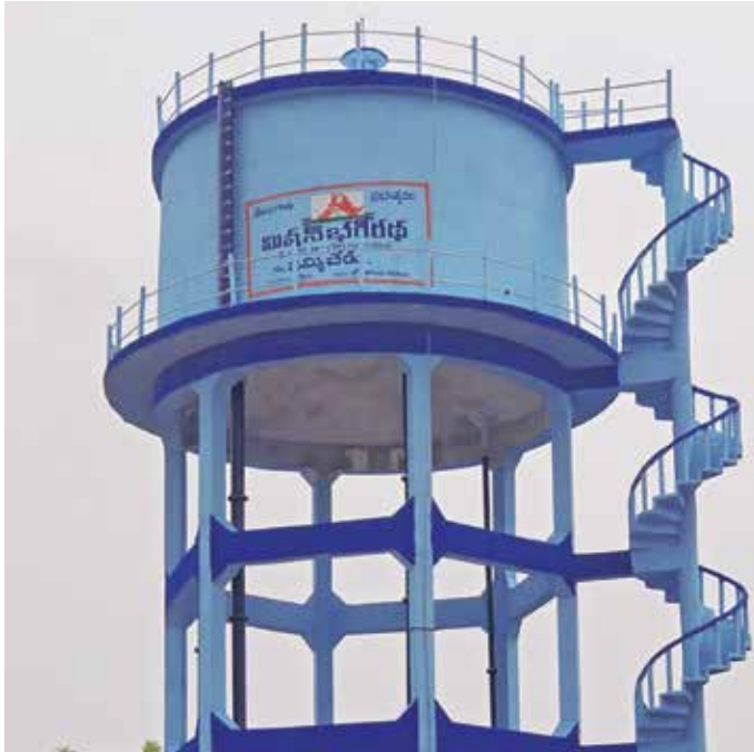
120 KL x 12 Meter Staging OHBR at Jammichedu for Jurala (TDWSP) Project, in Telangana.
