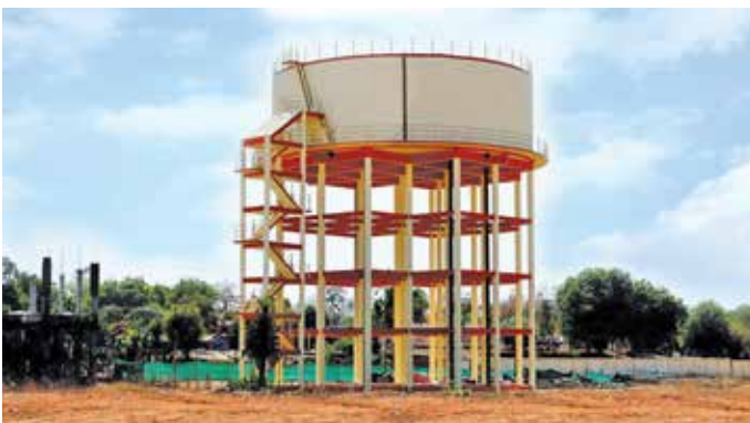
2,000 KL OHBR at Kushmonda for Guna Water Supply Project, in Madhya Pradesh.
