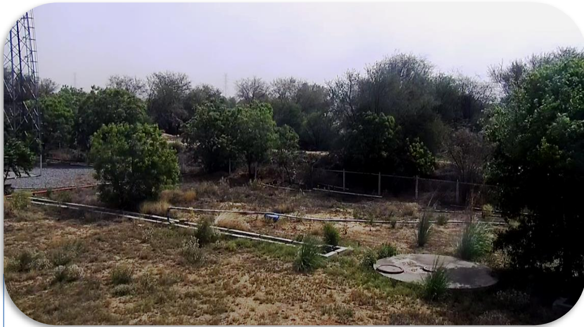
Rainwater harvesting system
