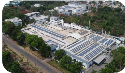
Ajanta Manufacturing Facility – Paithan, Aurangabad
