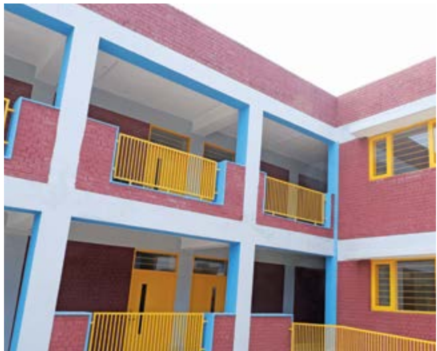
Outside view of Government High School, Giaspura (Pb)
