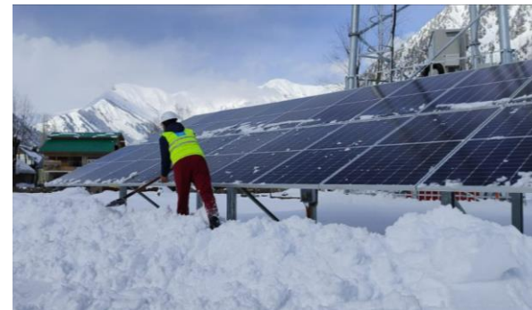
Site operations during heavy snowfall
