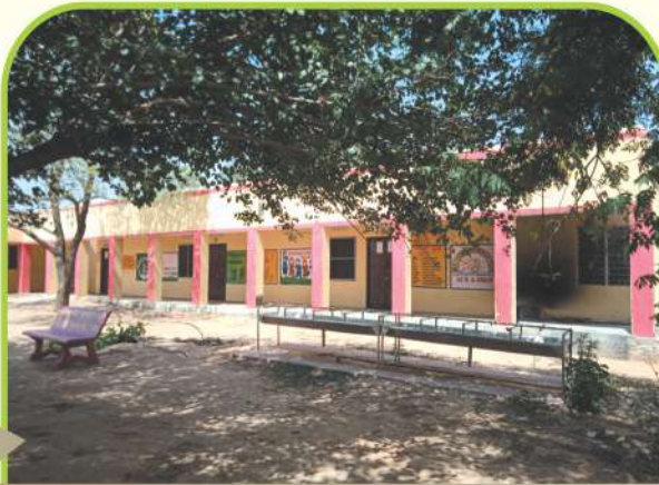
Installation of Hand Wash Station at Various Govt. Schools
