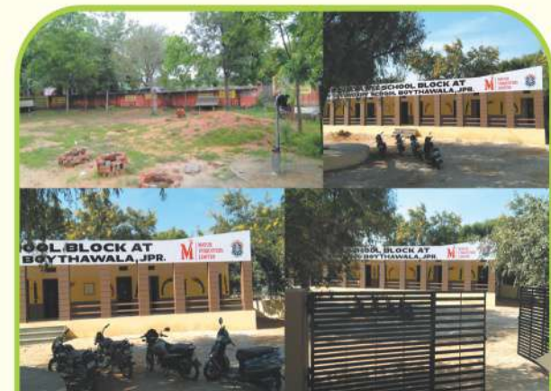
Renovation of Govt. School, Boythawala
