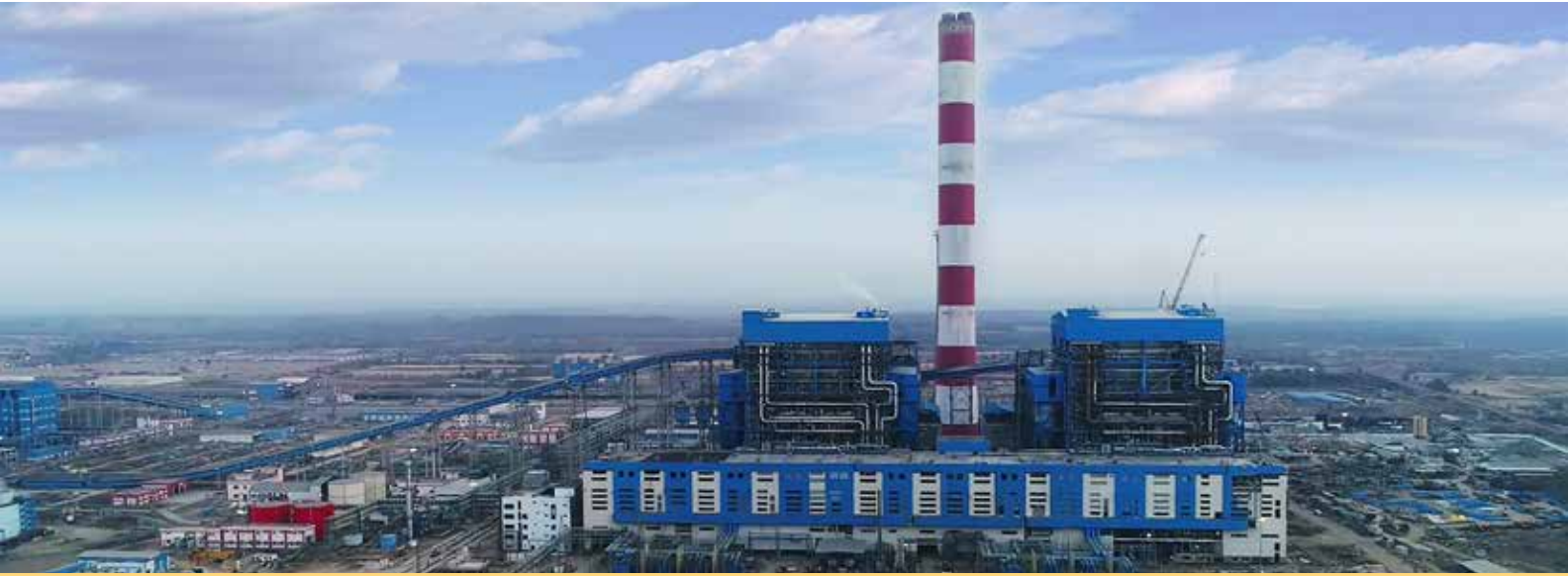
Flue Gas Desulphurisation (FGD) system at India's first ultra-supercritical thermal power plant, Khargone, Madhya Pradesh
