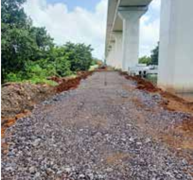
Approach road using steel slag
