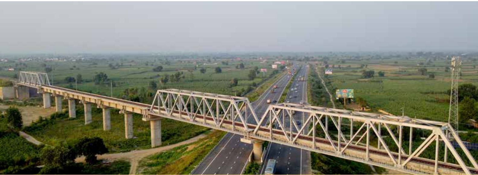
Eastern Dedicated Freight Corridor (Contract Package 303), Uttar Pradesh
