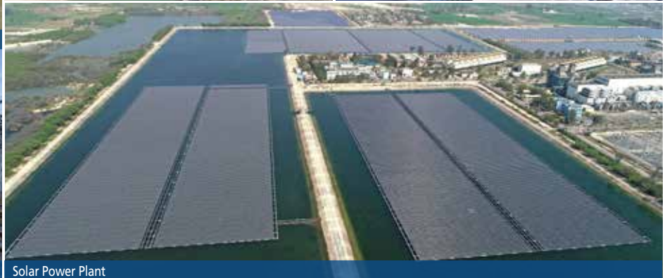
Solar Power Plant
