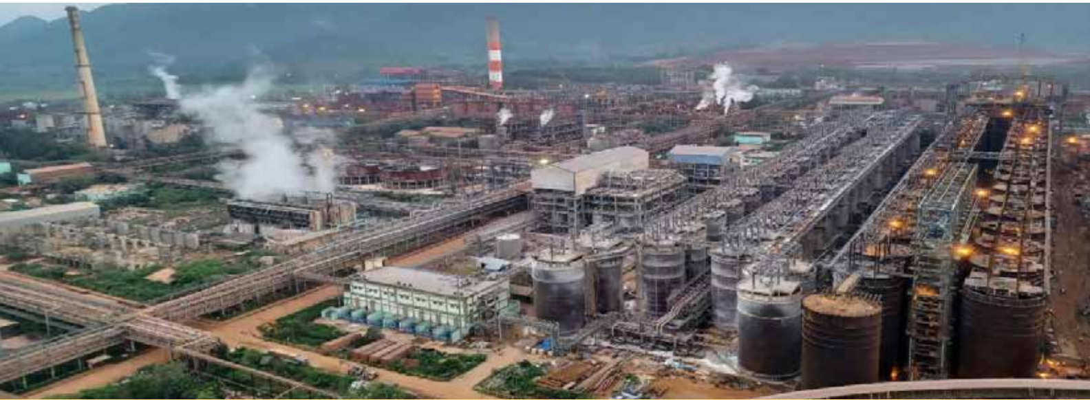
Alumina Refinery Expansion Project at Vedanta Lanjigarh, Odisha
