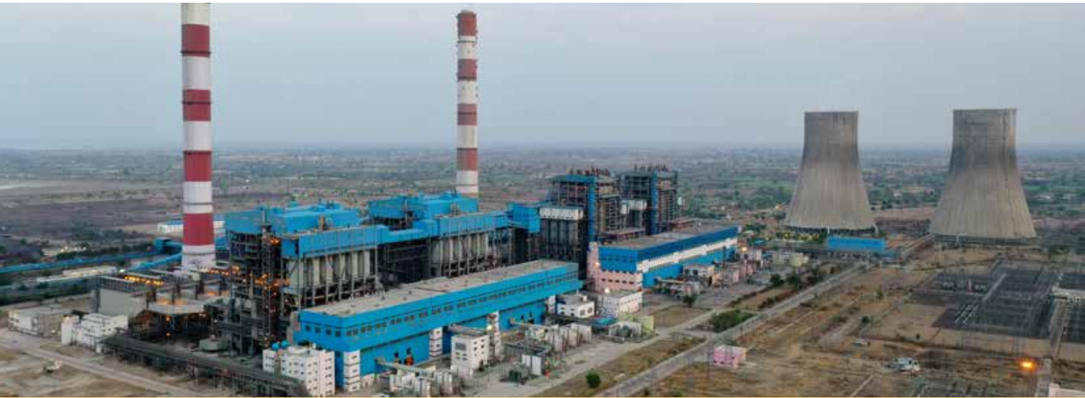
2x660 MW Shree Singaji Thermal Power Plant (Stage-II), Madhya Pradesh
