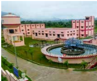
Water Treatment Plant
