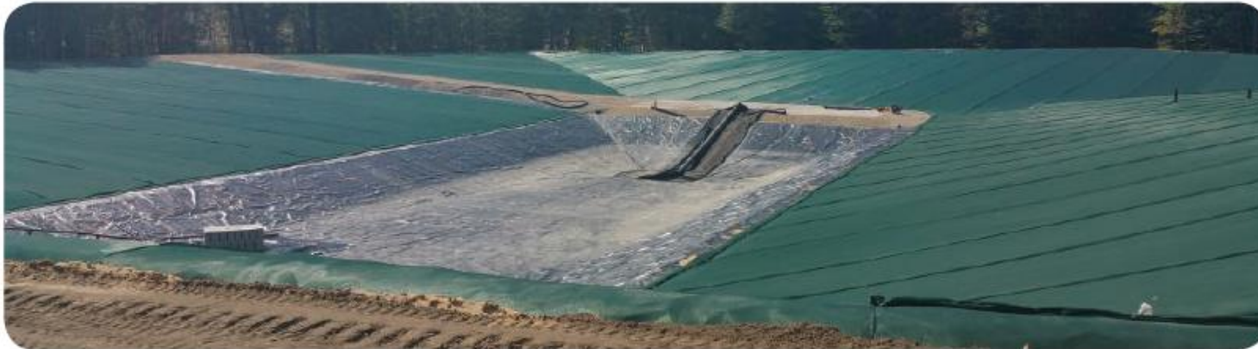
Leachate Spray Curtain - 262,400 sq.ft.
