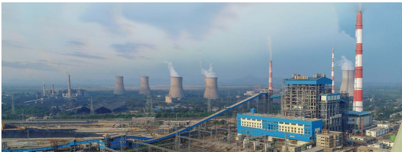
Kothagudem Unit 12 (800MW) commissioned by BHEL, achieved highest PLF of 85.5% and OA of 94.4%, among BHEL supplied supercritical sets
