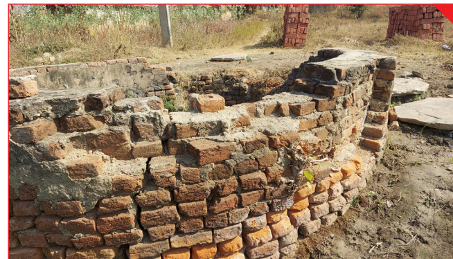
Condition of wells prior to JMFF intervention
