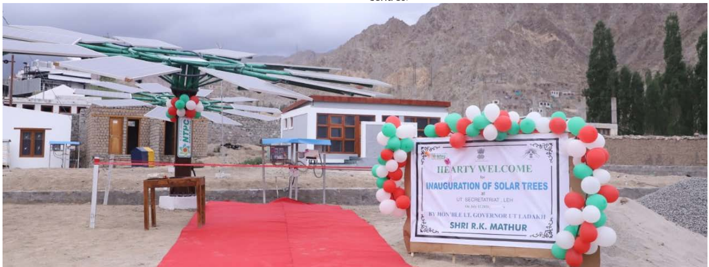
NTPC Solar Trees at Leh
