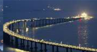
Hong Kong–Zhuhai– Macau Bridge
