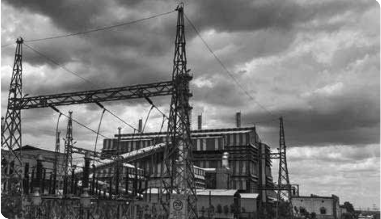
Newly Commissioned Ferro Alloys Plant
