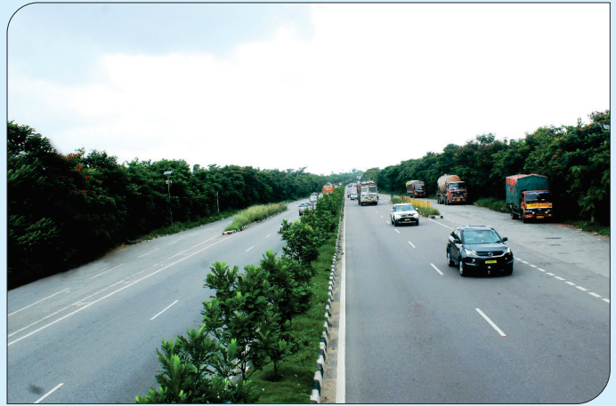
HKR Roadways Limited
