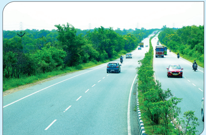
HKR Roadways Limited
