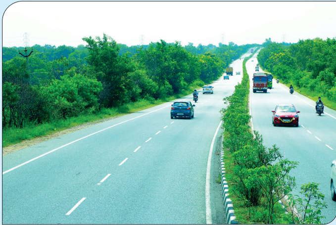
HKR Roadways Limited
