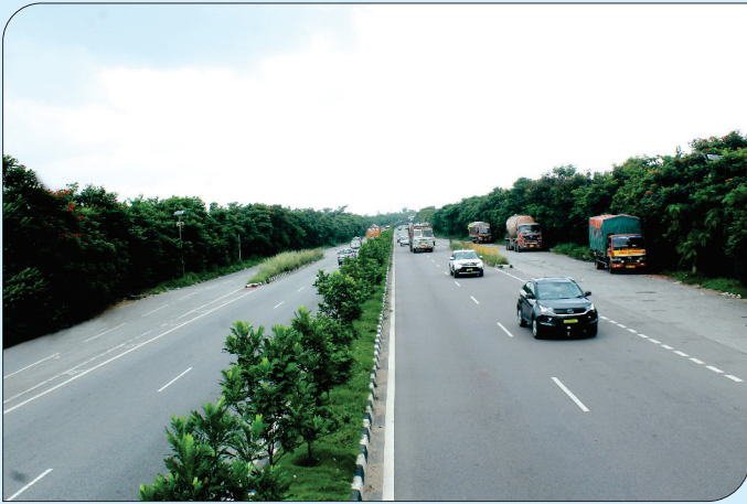
HKR Roadways Limited
