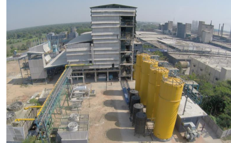
Multiple Effect Evaporator Plant (MEEP)
