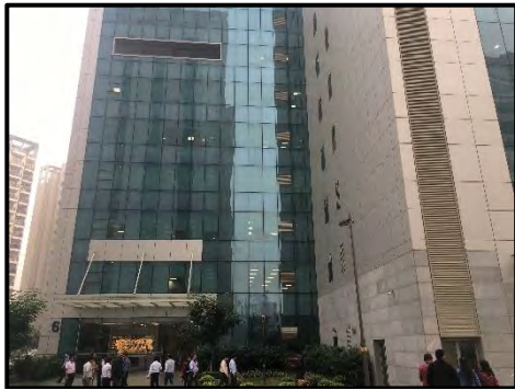
View of Tower 6
