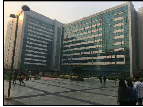
View of Tower 2 & 3
