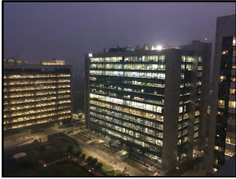
View of Tower 1
