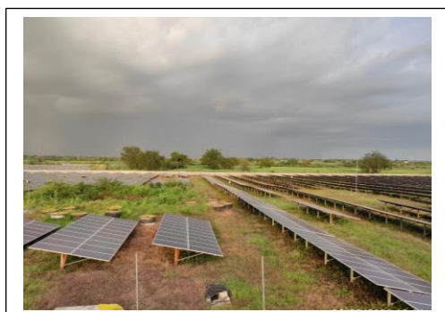
External view of the subject property
