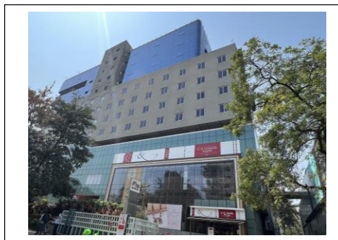
Building B (Center I)
