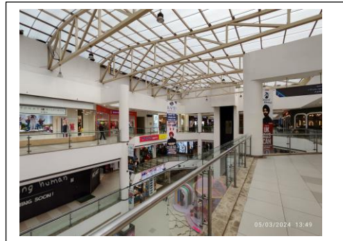
Internal view of the subject property
