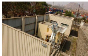
Waste Water Treatment Plant
