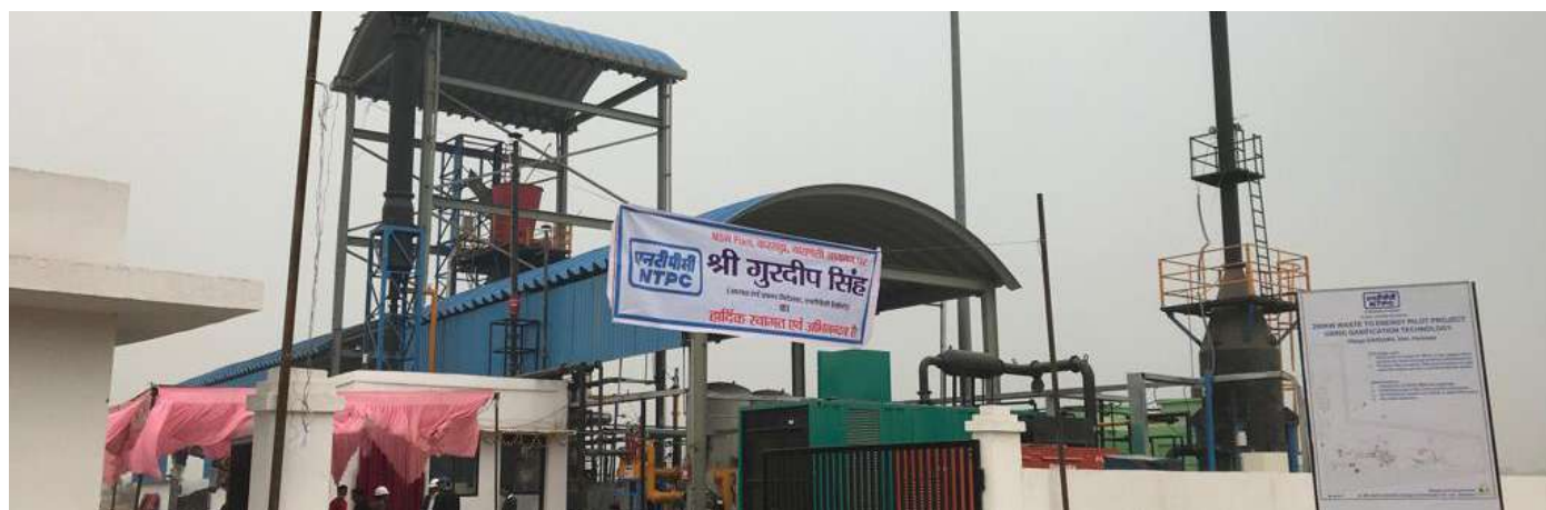
Waste to Energy Plant, Varanasi
