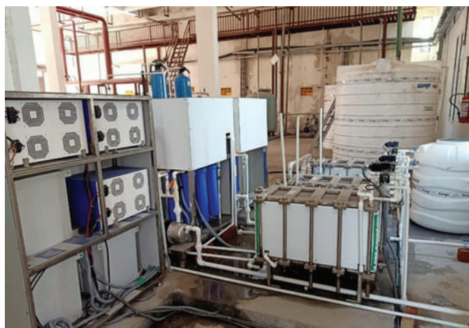
24 TPD Electro-Dialysis Reversal (EDR) Plant, NETRA
