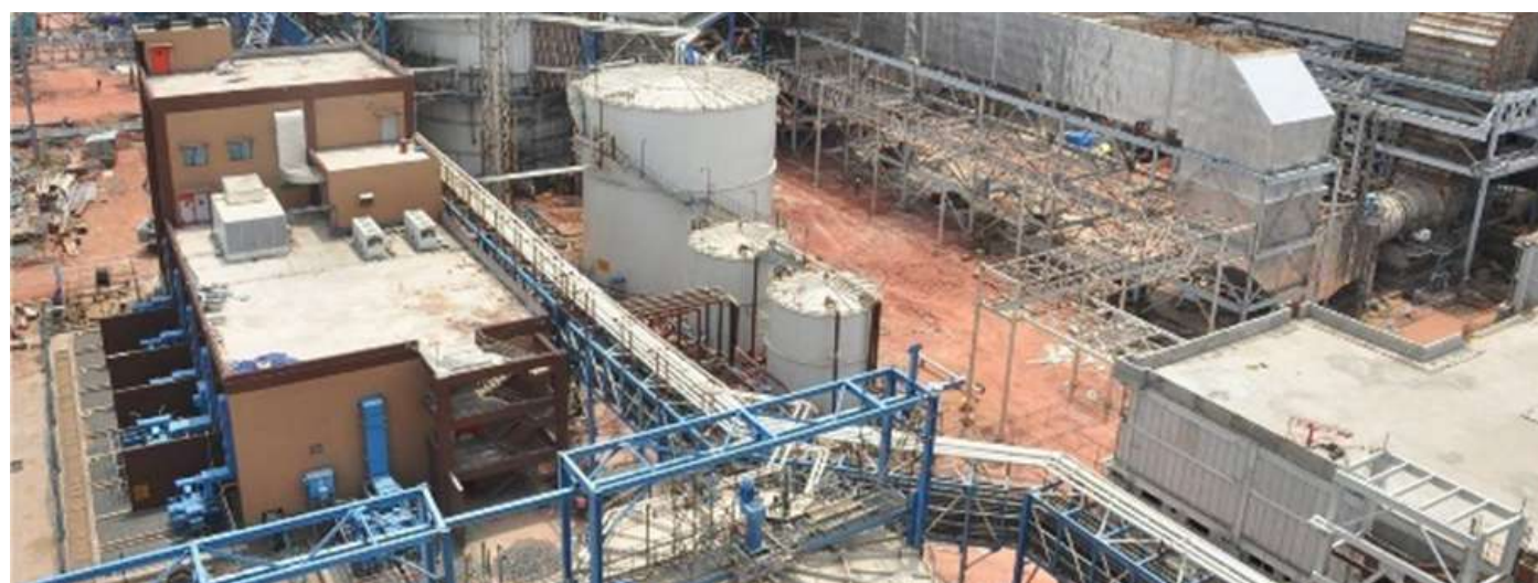
FGD Installation at NTPC, Telangana
