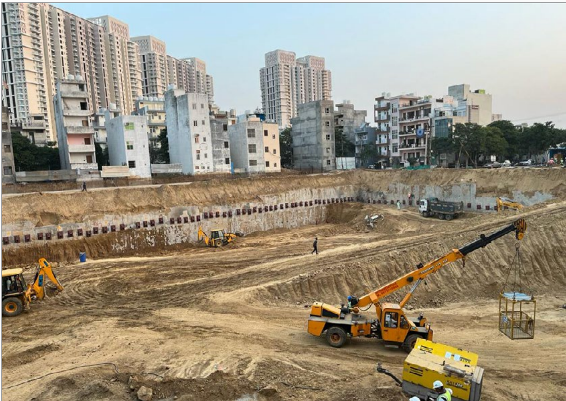
Summit Plaza, DLF5 under construction in Gurugram
