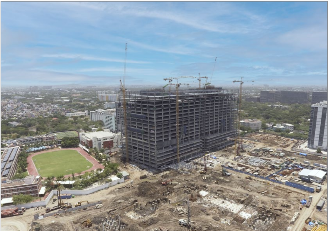
DLF Downtown under construction in Chennai
