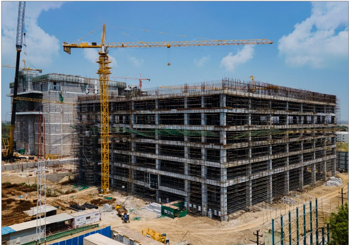
DLF Tech Park & Data Center under construction in Noida
