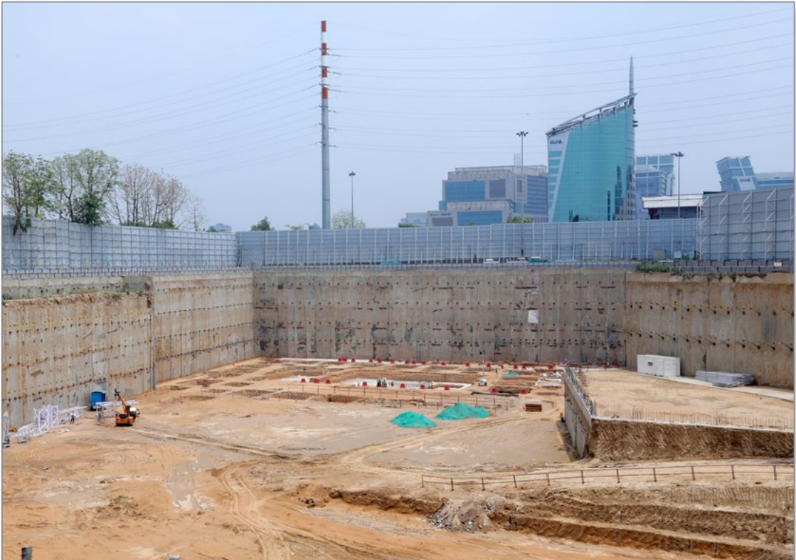
Atrium Place under construction in Gurugram
