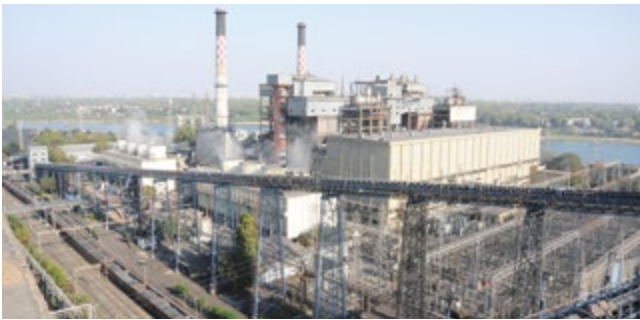
362 MW AMGEN Power Plant at Ahmedabad
