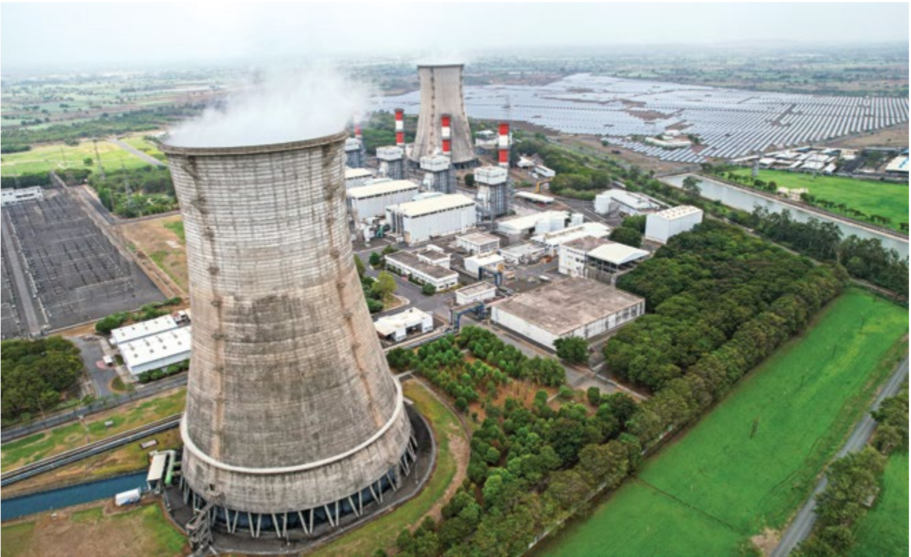
1,530 MW SUGEN & UNOSUGEN Plant at Surat
