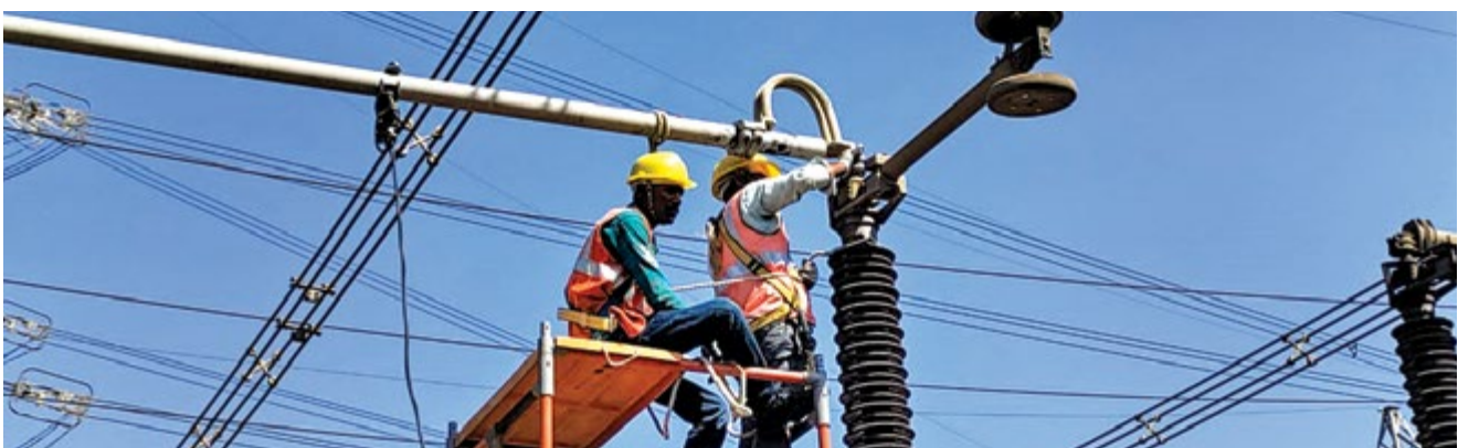
Use of safety suits during work execution
