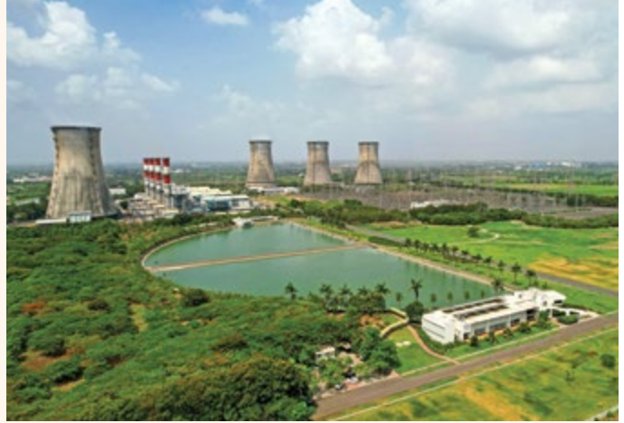
1,530 MW SUGEN & UNOSUGEN Plant at Surat
