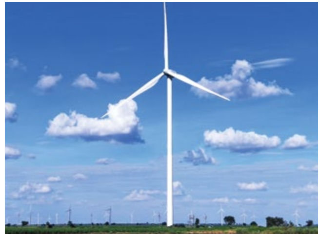
120 MW Gamesa Wind Power Plant at Karnataka
