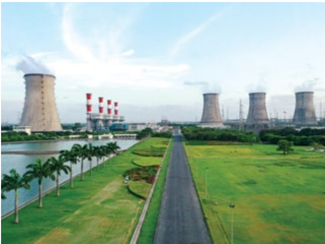
1,530 MW SUGEN & UNOSUGEN Plant at Surat
