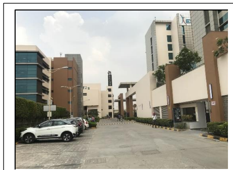
View of internal road
