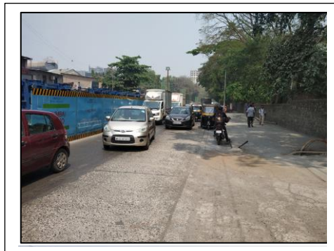
View of the primary access road/entrance
