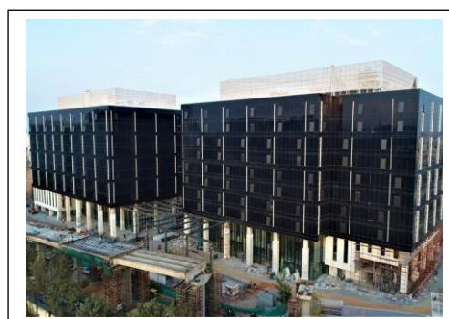
View of recently completed NXT block
