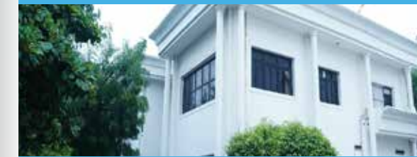
State-of-the-art D9 US FDA accredited API facility at Panoli, Gujarat
