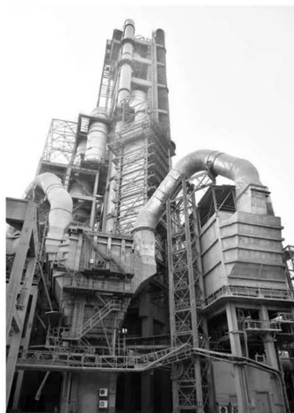
5 stage Pre Heater and Electrostatic Precipitator (ESP)
