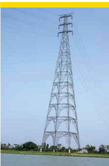
400 kV Ashuganj-Bhulta Transmission Line; tallest transmission towers in Bangladesh
