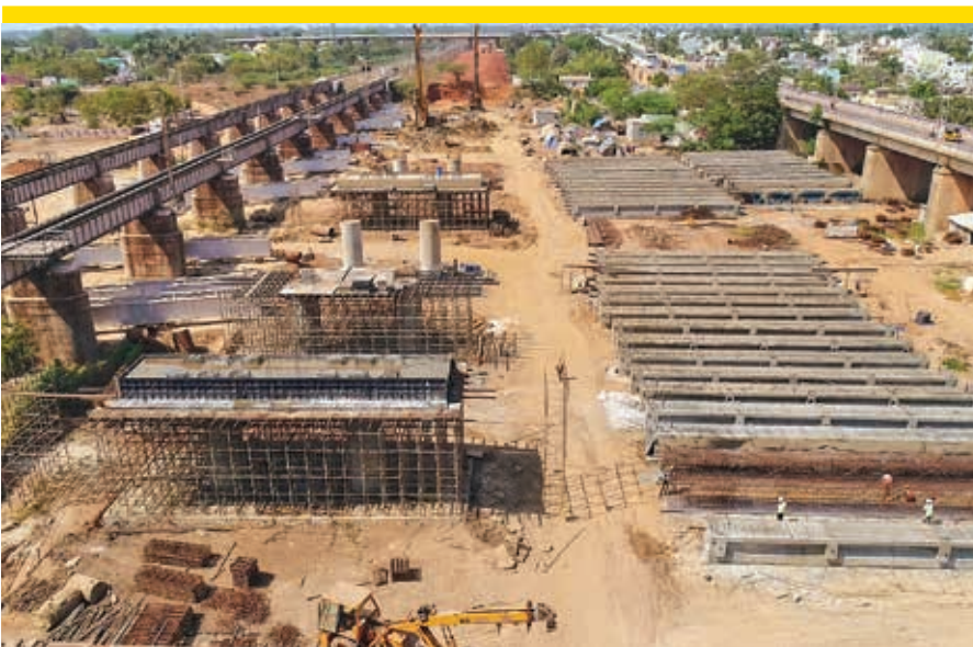
Work at major bridge across river Penna
