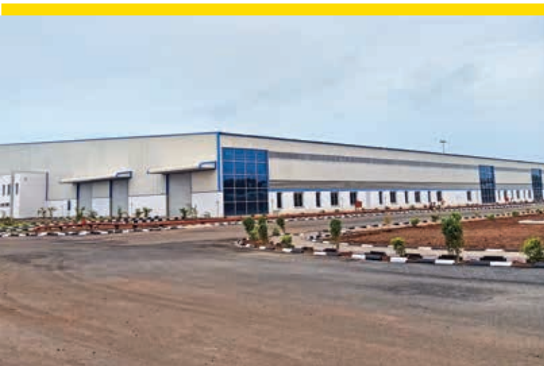
Manufacturing facility for an automobile manufacturer, Andhra Pradesh
