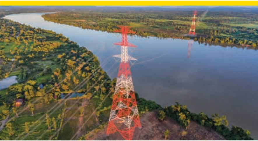
500 kV Thai Lao Border-Ubon Ratchthani Transmission Line, Thailand
