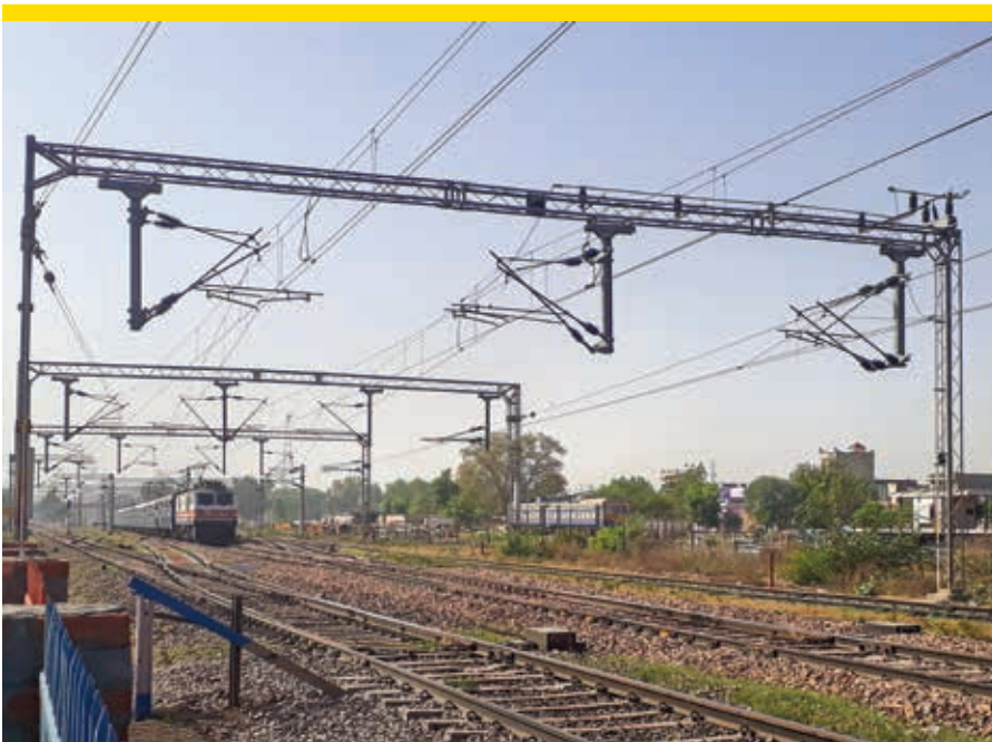
Electrification of 85 RKM section between Narwana to Kurukshetra, Haryana
