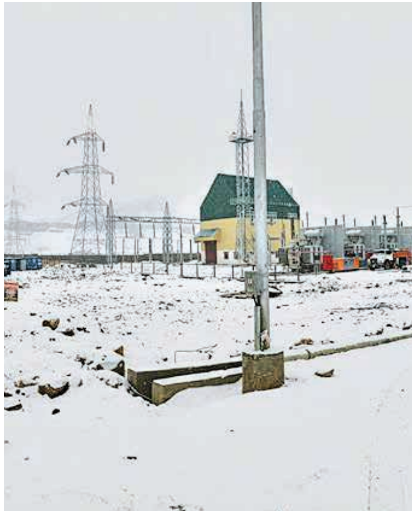
220/66 kV GIS Substation at Drass, Jammu & Kashmir; second coldest inhabited place on Earth
