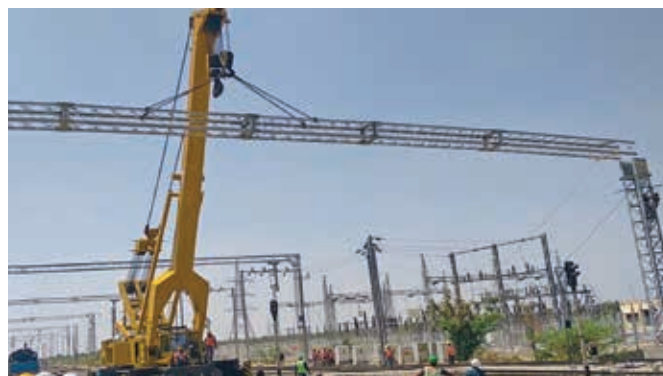
Erection of a complex Boom structure in Ajmer-Rani Railway Electrification project
