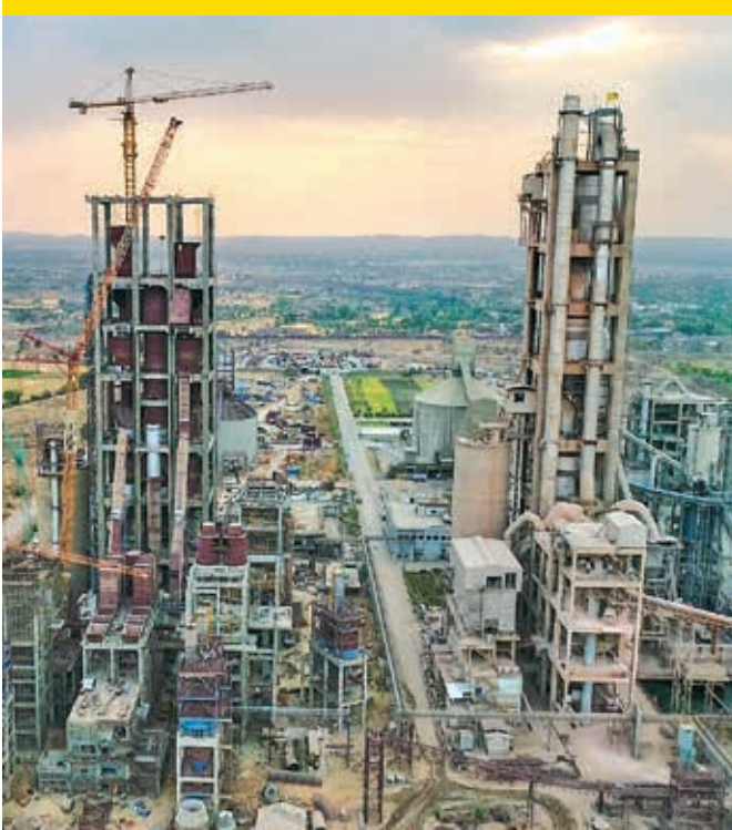
136m tie-beam at brownfield cement manufacturing plant, Rajasthan
