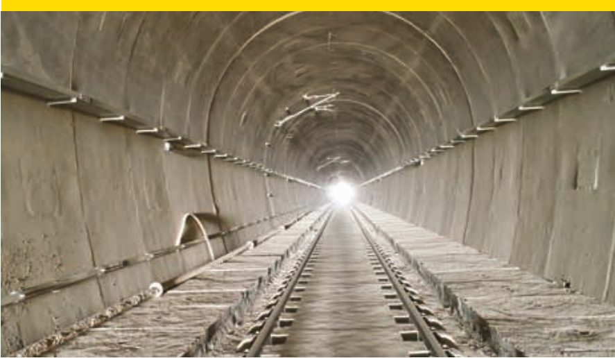
Electrification works of India's third longest railway tunnel
