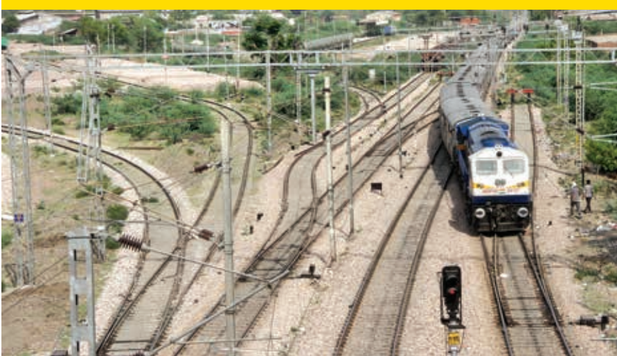
Railway Overhead Electrification between Mathura-Achnera Uttar Pradesh/Rajasthan
