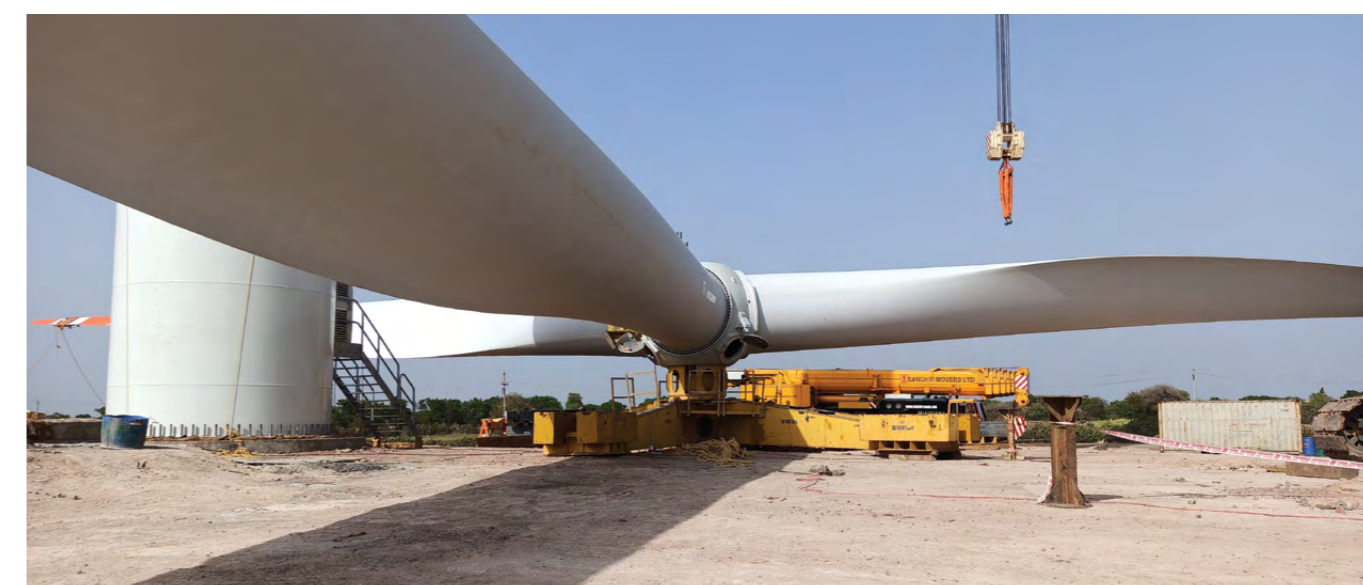
115 MW SECI-V Wind Power under construction Project, Jam Khambhalia, Gujarat
