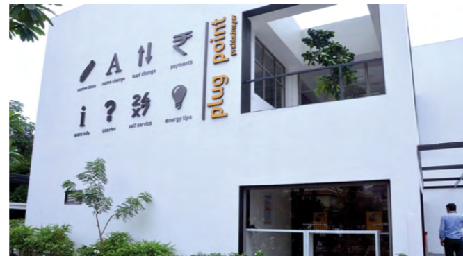
State-of-the-Art Plug Point at Ahmedabad
