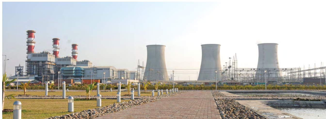
1,200 MW DGEN Power Plant, Dahej
