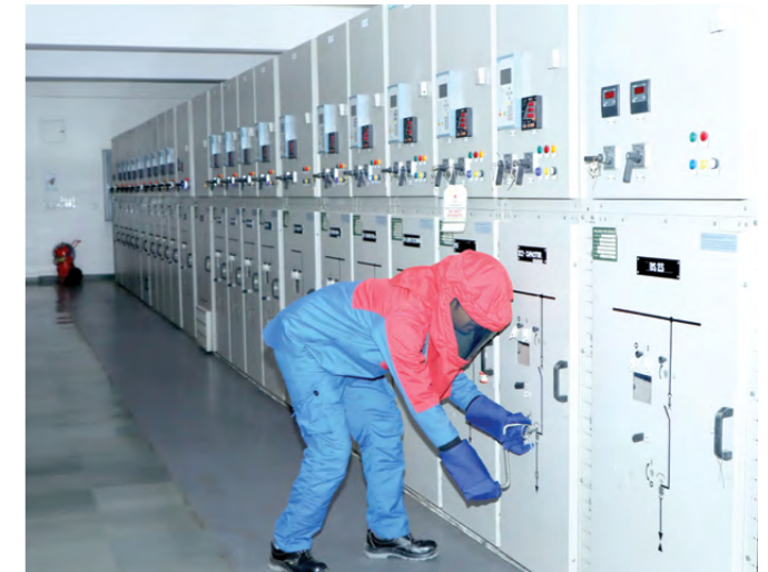
Use of Arc Suit during EHV Operations
