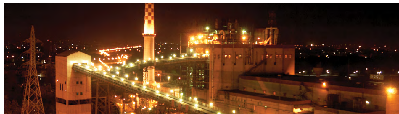
362 MW AMGEN Power Plant, Ahmedabad
