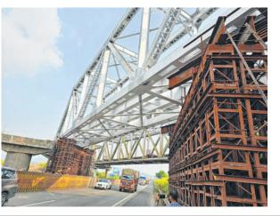
minutes before the targeted time of 5pm. The successful launch of the girder, weighing 250 metric tonne, over the Pune-Mumbai Expressway was achieved with utmost precision and adherence to safety protocols," he said.
