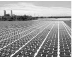
file photo of a floating solar power plant at an NTPC unit
