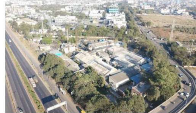
Our Ankleshwar Facility - Gujarat
