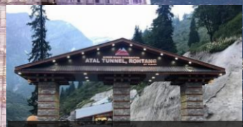
Atal Tunnel, India
