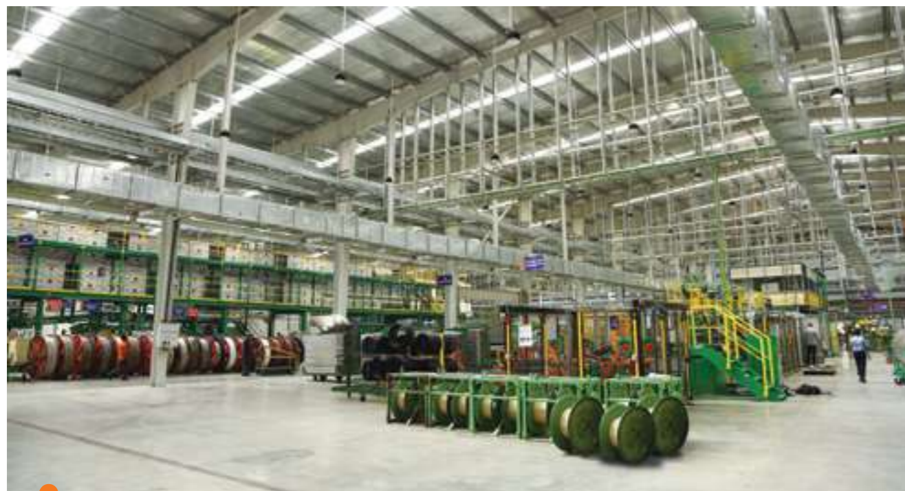
Manufacturing Plant at Halol
