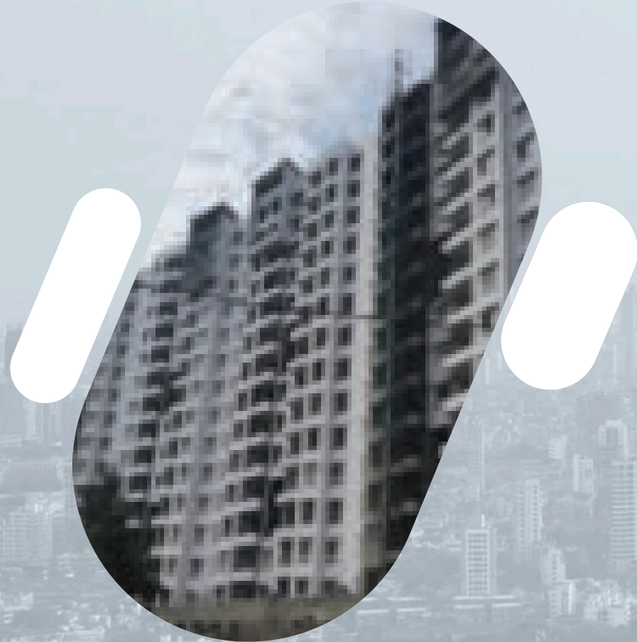
Actual site status on 30th September
