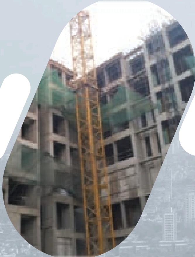
Actual site status on 30th September
