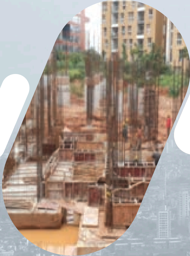
Actual site status on 30th September
