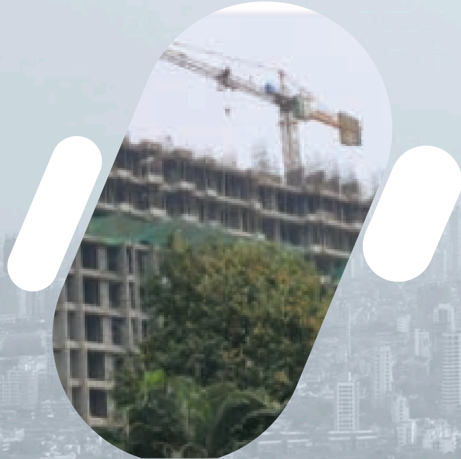
Actual site status on 30th September
