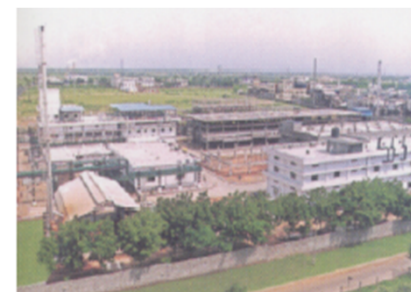
SUVEN Intermediate Mfg. Facility, Suryapet, India
