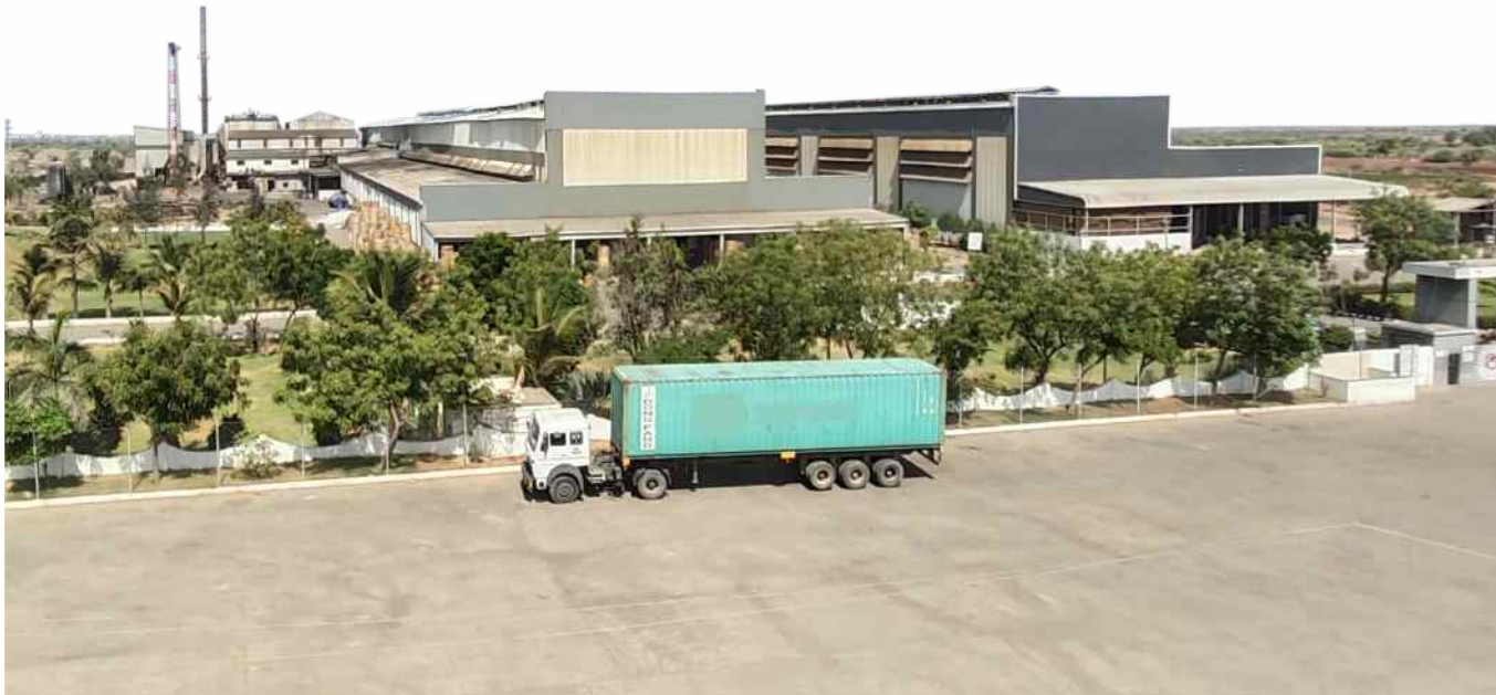
UNIT-1 HALVAD PLANT (GUJARAT)
