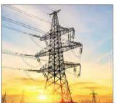
■ The action has been taken under the Electricity (Late Payment Surcharge and related matters), Rules 2022
