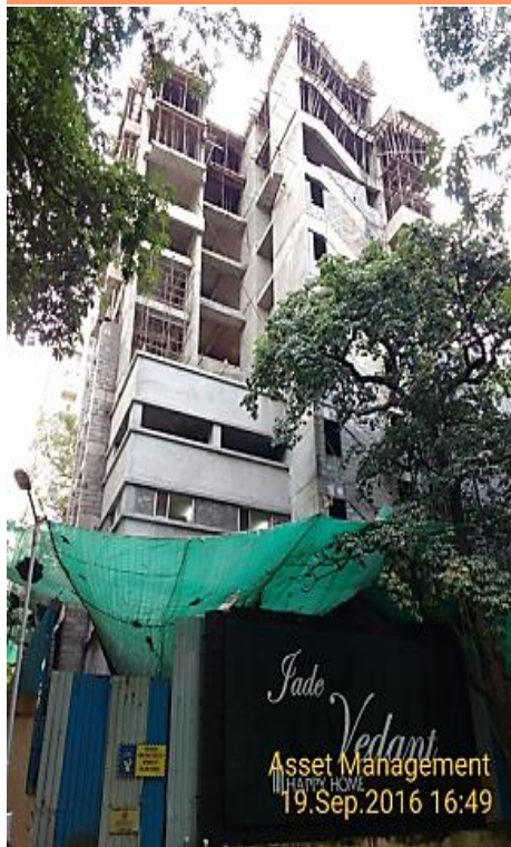
Sep'16 – 5 th Floor completed
