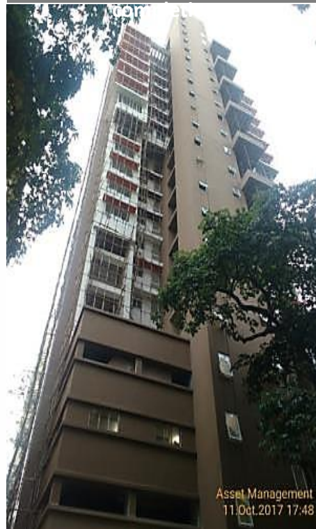
Oct'17 – Finishing near
