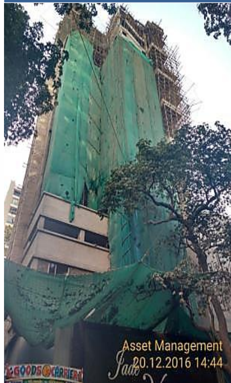
Dec'16 – 9 th Floor Completed
