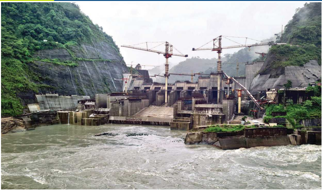
2000 MW Subansiri Lower Project (Arunachal Pradesh/ Assam) - Dam under construction
