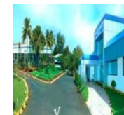
KSB MIL Controls Ltd. Meladoor, Kerala
