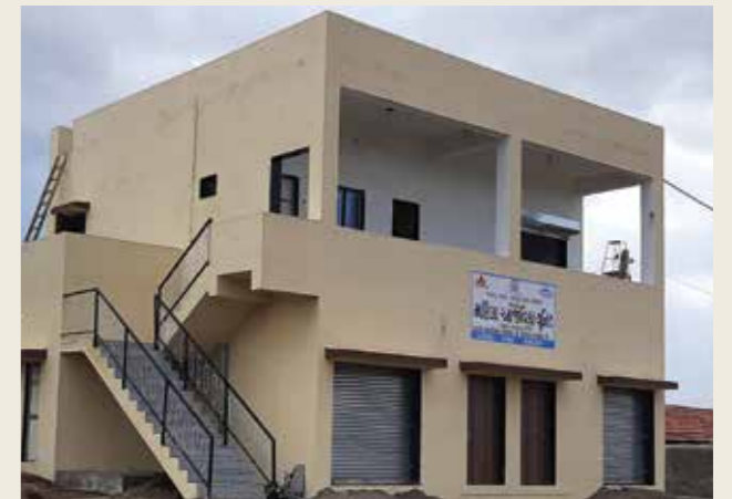
New SHG units being constructed
