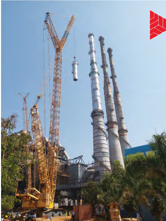
In Rayagada, LR1750 (750 MT Crane) busy in stack erection
