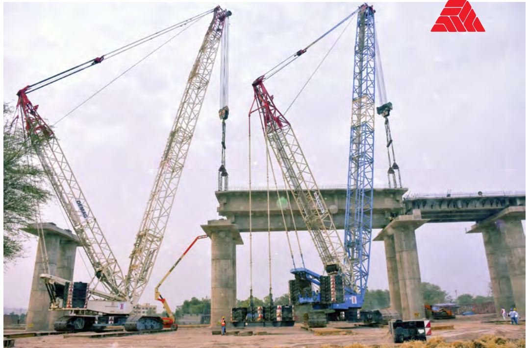
Girder erection in tandem lifting with 2 x CC2800-1 (600 MT Crane) - at Sohna Project
