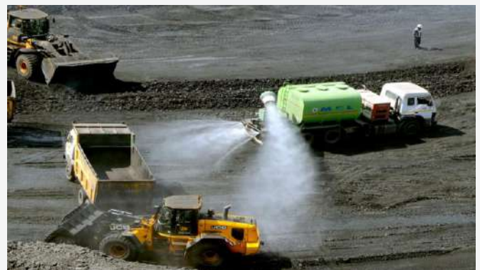
Fig. - Mobile Fog Canon in operation for suppression of dust at the source
