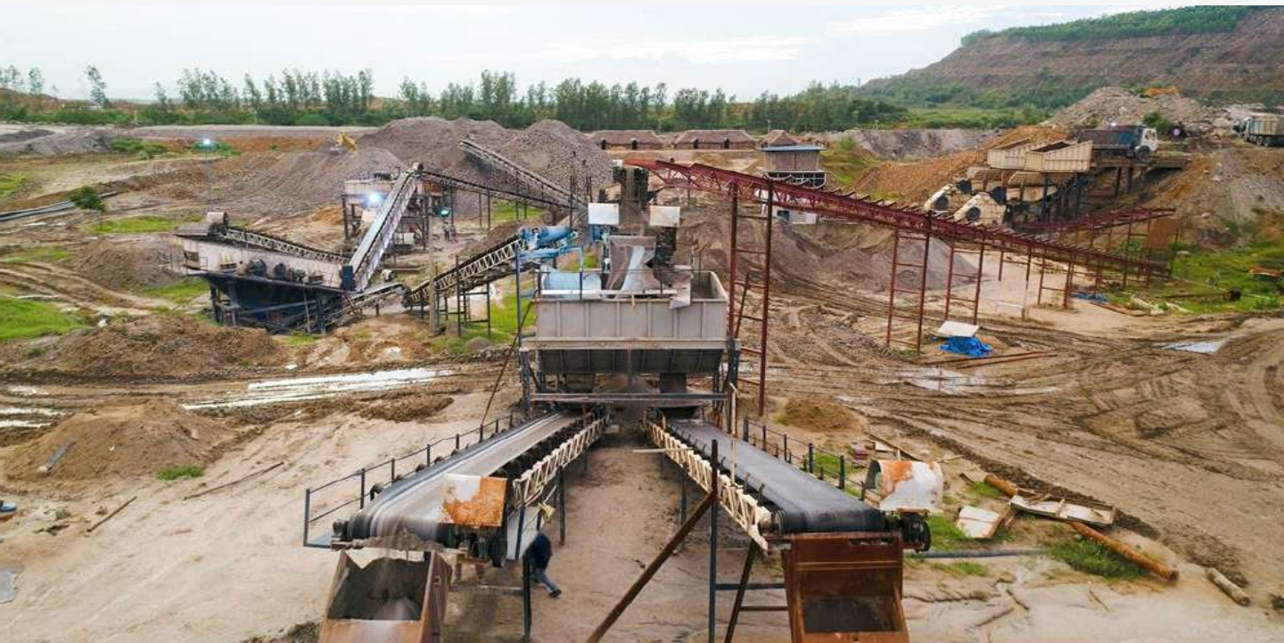
Fig. - OB to sand plant in WCL
