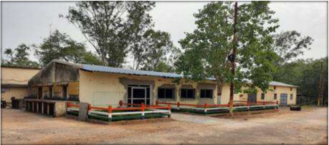
Fig. - Exterior View of under-construction museum
