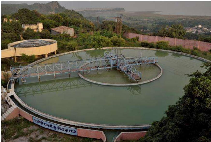
Fig. 55-Water Treatment Plant in NCL
