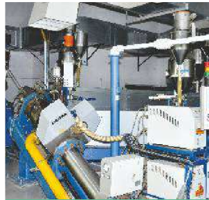
550 kV Mallefer HVCV Insulate Line
