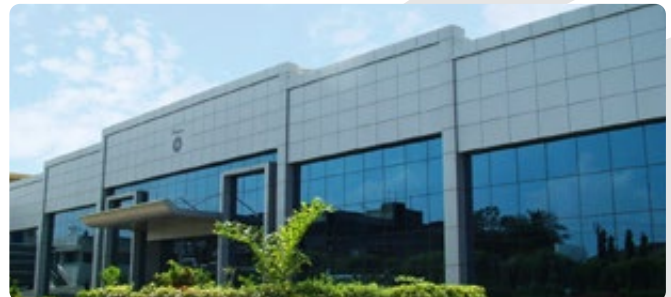
State-of-the-art Tablets and Lozenges manufacturing facility at Kadaiya, Daman
