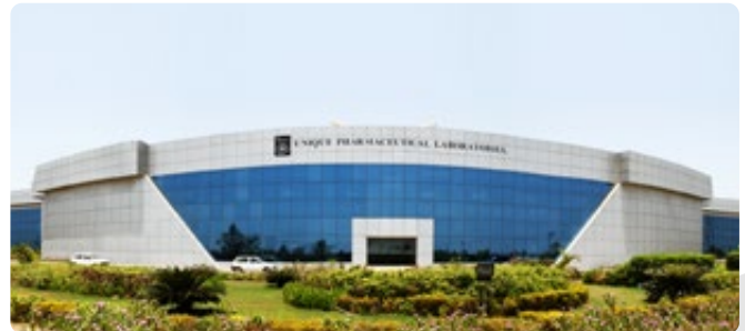
State-of-the-art Formulations manufacturing facility at Panoli, Gujarat
