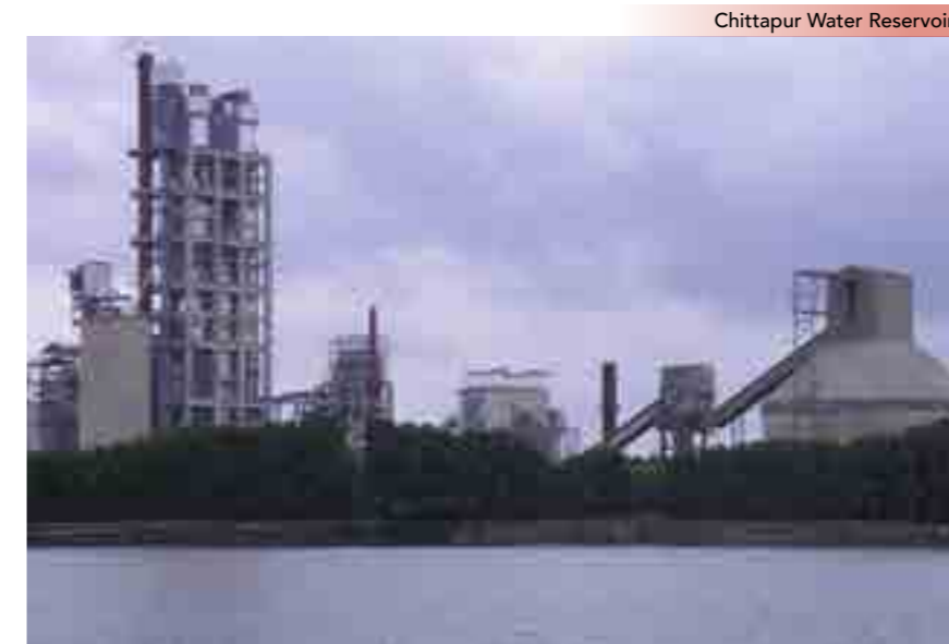
Chittapur Water Reservoir
