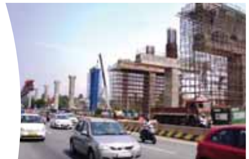
Erected Viaduct & Station Works under construction for Bangalore Metro Railway Project
