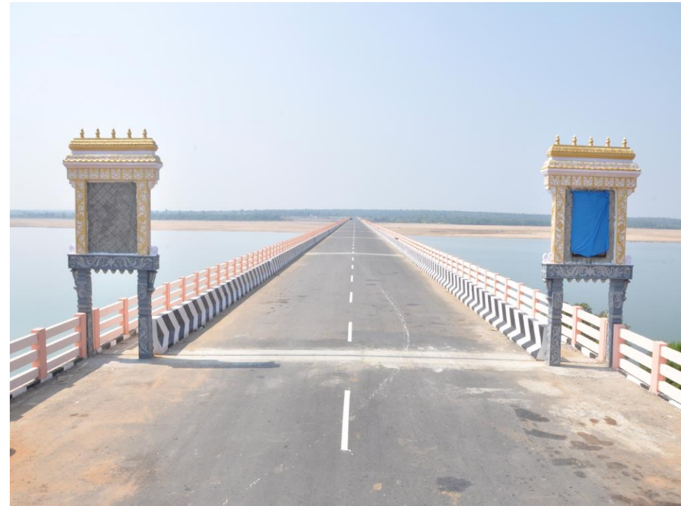
Eturunagaram Bridge over river Godavari
