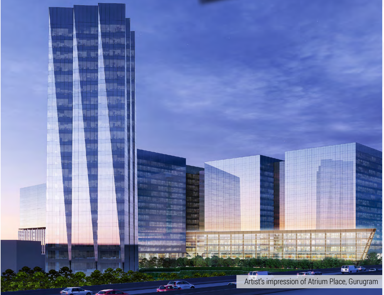
Atrium Place, Gurugram under construction
