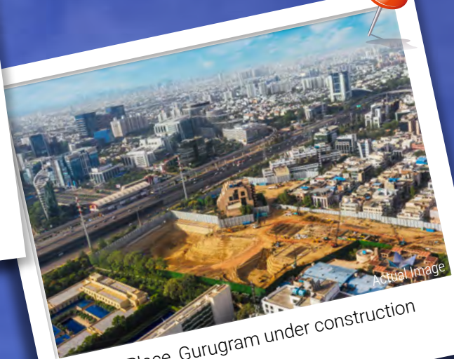
Atrium Place, Gurugram under construction
