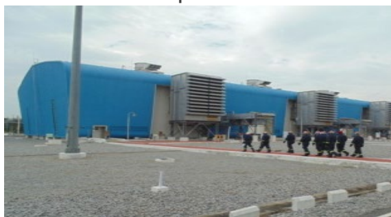
CS - 3 Compressor House
